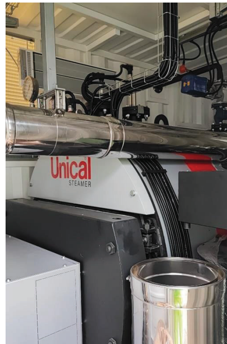
Fig. 9 – steam generator – container and steamer
